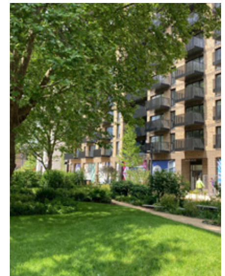
Figure 5.42: Well articulated façades with balconies and large openings will provide natural surveillance to the gardens
