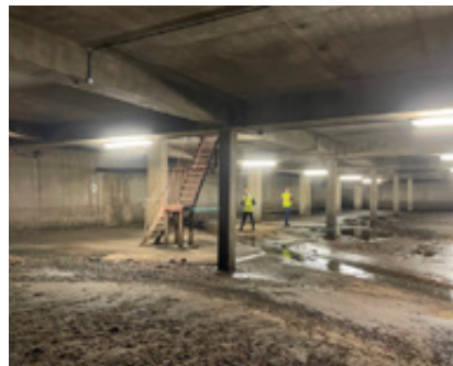
Figure 6.4: Thames Water attenuation tank in the basement of the car park
