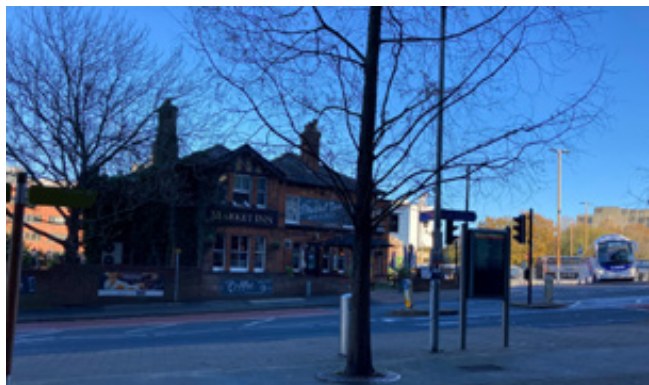
Figure 3.5: Market Inn - Locally listed
