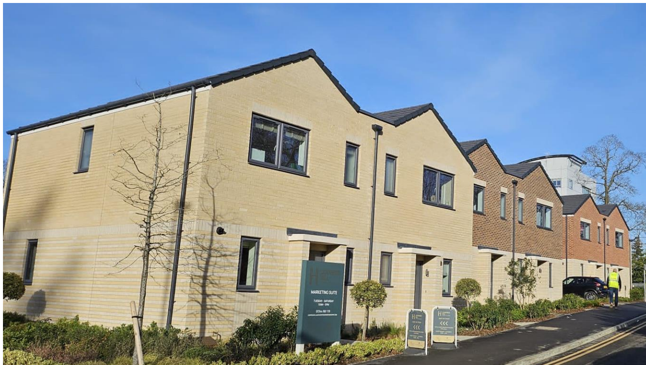
Figure 2. Coopers Hill – Crowthorne Rd Marketing Suite & completed new homes
