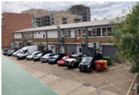
Figure 6.3: Existing service area at the rear of Market Street
