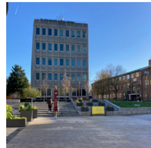
Figure 7.28: Easthampstead House and Town Square as viewed today on approach from the town centre along The Avenue
