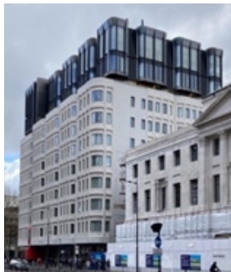
Figure 7.21: Easthampstead House can be refurbished and extended at roof level with terraces providing long distance views, example: ex Camden Council Office, London
